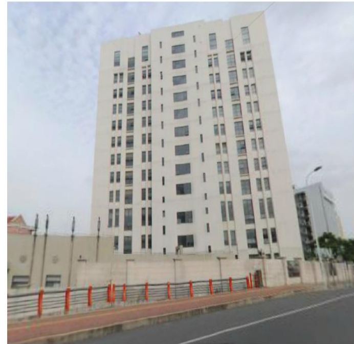
FIGURE 7: Unit 61398 Center Building 208 Datong (rear view, possible generator exhausts visible) Image Copyright 2013 city8.com
